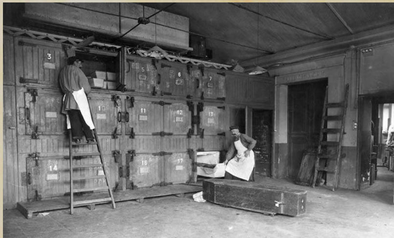
Morgue room of fridges at the beginning 20 th
