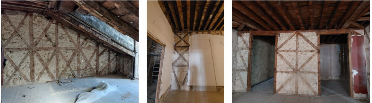
Figure 38 –From left to right , frontal walls at roof level; front walls on levels below (Pictures taken on site)
