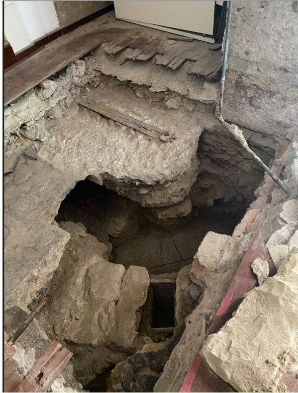
Figure 31 – Trial pit to the existing foundations at lower ground floor (Picture taken on site)
