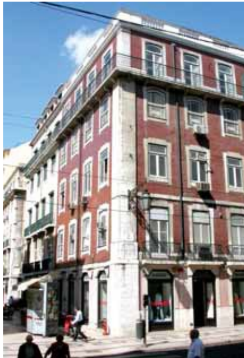
Figure 24 – Example of a building with Pombalino Façade that has been extended with Gaioleiro type construction Rua da Assunção 34-40 Lisbon (Image from (Lisboa, 2005))
