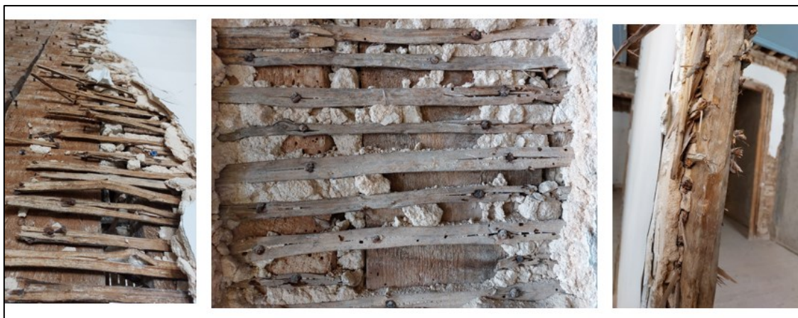
Figure 37 – Examples of “Tabique Walls” on site (Pictures taken on site)
