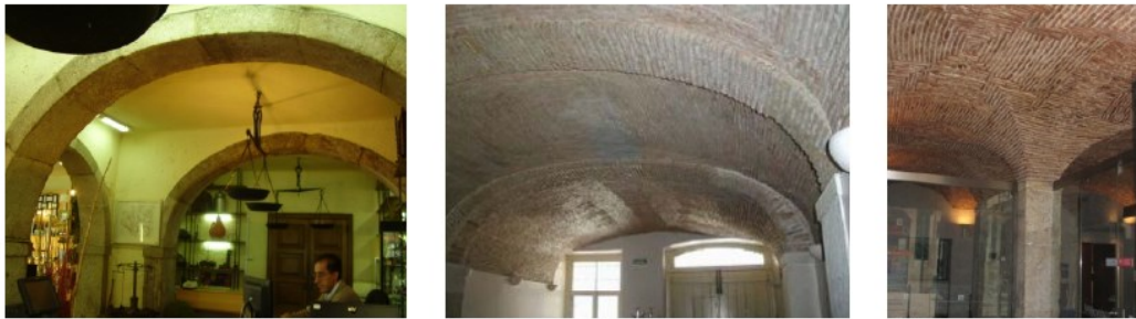
Figure 17 – From left to right: Solution of arches and beams, Barrel vaults made in masonry, crossed vaults made in masonry (Simões & Bento, 2012a)
