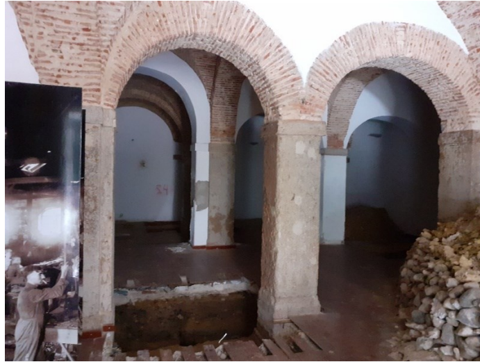
Figure 34 – Columns in contact with the ground made of stone masonry (picture taken on site)
