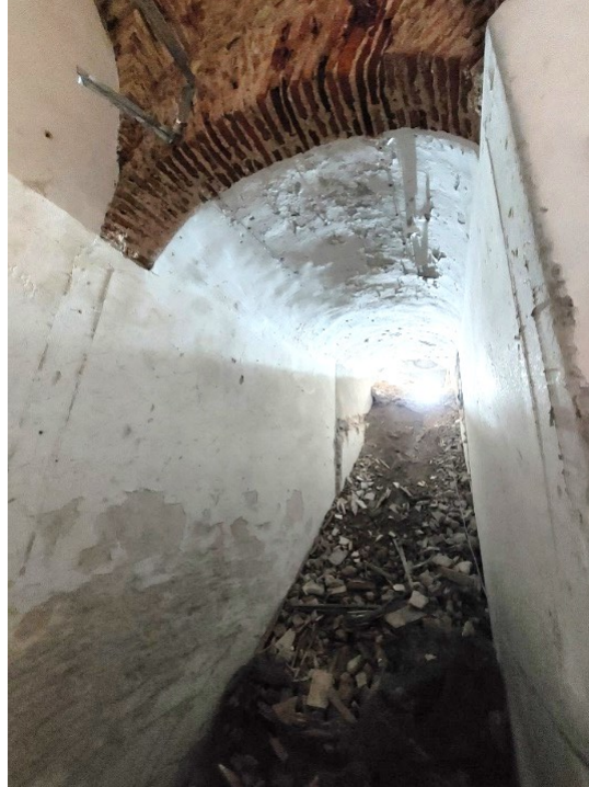
Figure 33 – Tunnel access from ground floor at Rua do Alecrim to lower ground floor at rua das flores
