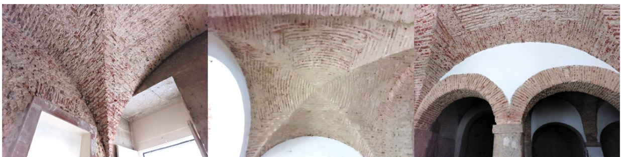
Figure 32 – Quadripartite Vault (Pictures taken on site)
