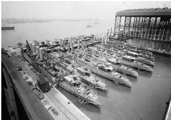
Figure 15 - This image of eight Wickes class destroyers, of the flush decker type, being built at New York Shipbuilding Corporation, Camden, New Jersey in 1919 illustrates the “quantity as a quality of its own” nature of the U.S. WW1 destroyer building program. Not an outstanding design, their availability in large numbers for conversion to oceanic escorts were to make them a vital weapon in the battle of the Atlantic in WW2.
