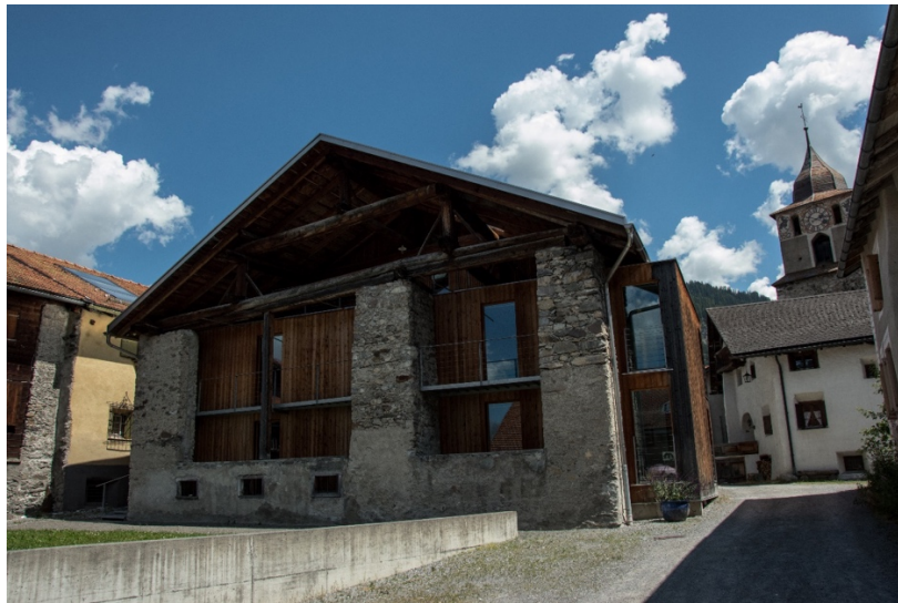
Figure 2. Danielle Marques and Bruno Zurkirchen, house in Bergün, 1994-1996. Wooden cuboid, wherein the residential function was inserted into the outline of the walls of the old barn, so that the windows are visible fragments of old walls. (source: author's photograph)
