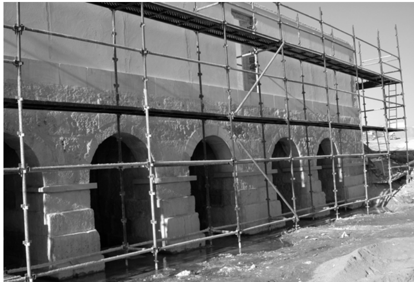
Figure 12: Montijo mill, Moinho do Cais (in restoration) – 2005
