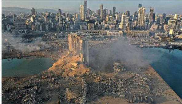
Figure 1 - Beirut Explosion Damage (Source: [3])
