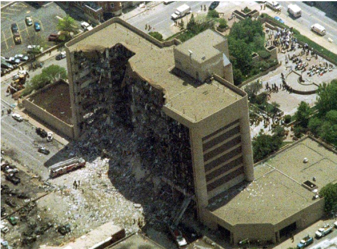
Figure 6 - Oklahoma City explosion damage (Source: [17])
