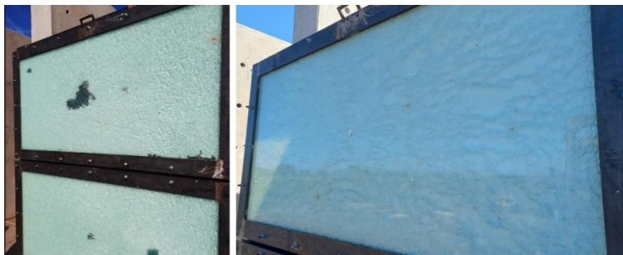
Figure 89 - Glass rupture pattern comparison, on the left failure due to impact, on the right failure due to shock wave damage
