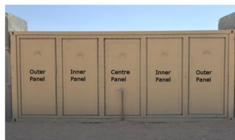
(b) ISO container made of front panels and a steel frame compliant.
