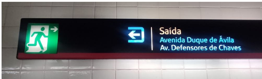
Figure 67. Signs indicating the direction to the emergency exit and the normal exit in the Lisbon metro at Saldanha station. All photos taken by the author, 2025.
