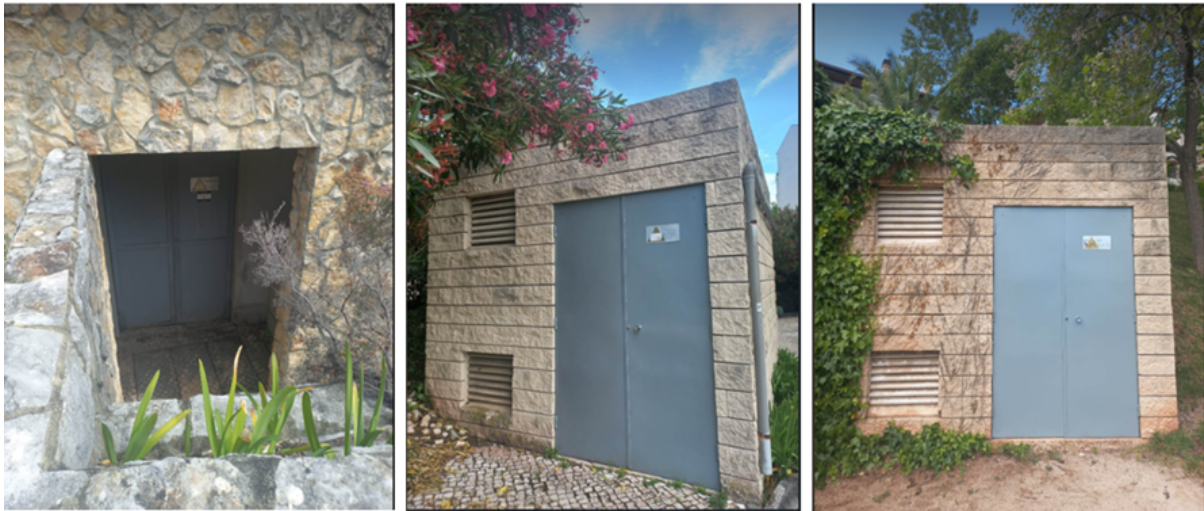
Figure 5.11: Access of the TS a) 662; b) 663; c) 664
