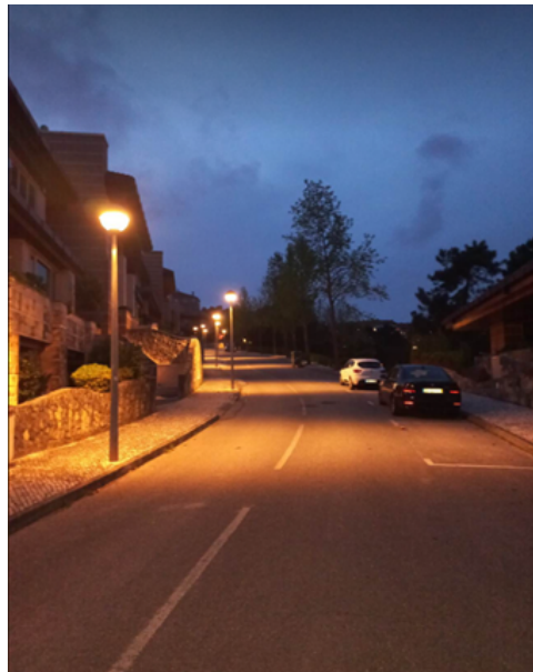
Figure 5.53: Poor overall uniformity
