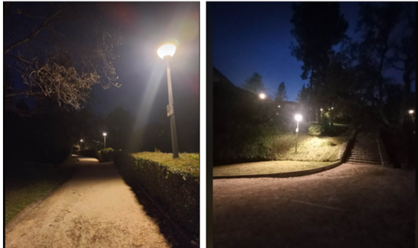
Figure 5.52: Poor lighting in pedestrianised areas
