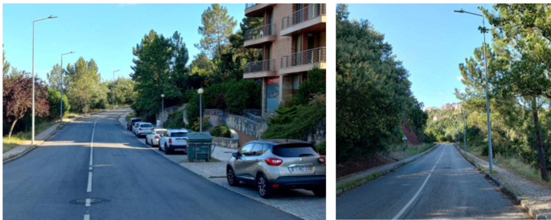
Figure 5.2: Edmundo Bettencourt Street I
