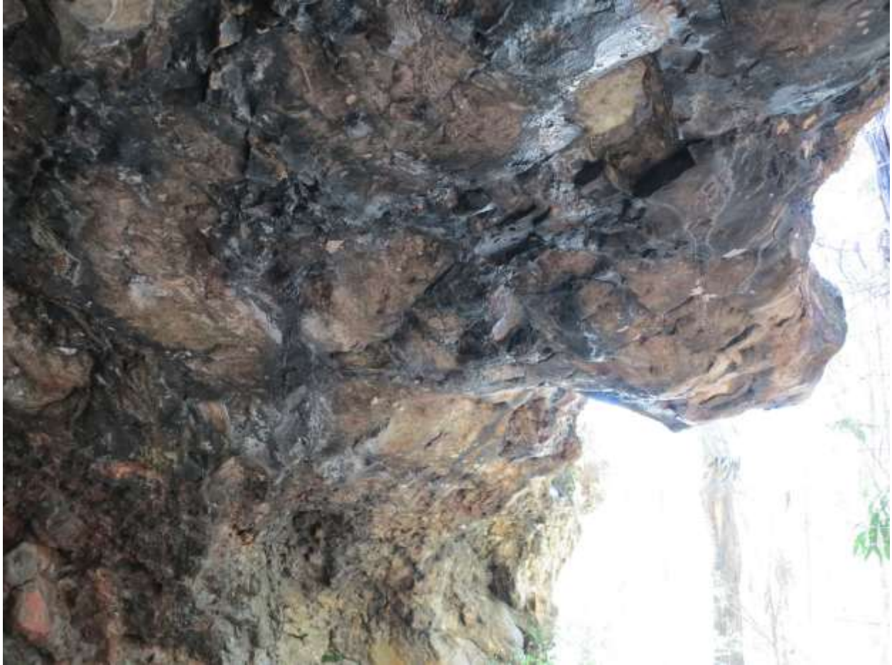
Figure 34 Impact of water percolating on the panels (Hipolito 2023).
