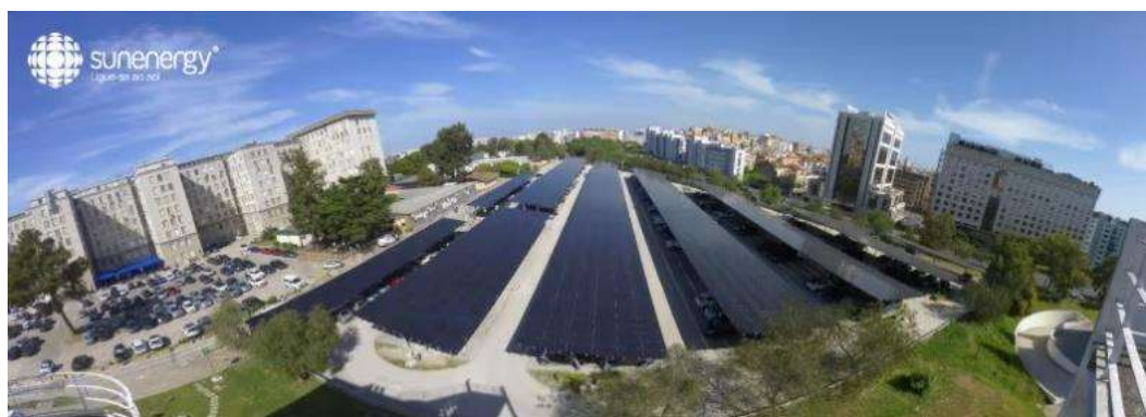
Figura 6.26 Carpark instalado no Hospital Santa Maria – Lisboa
