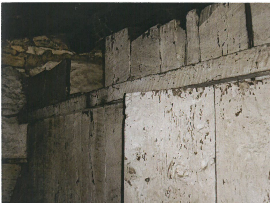
Fig.30 Divisória interior de taipal (Inq.05)
