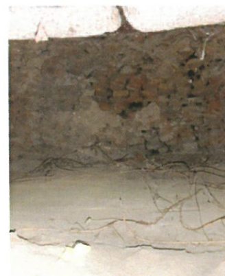
Fig.76 Interior "forno" tijolos de barro (Inq.14).
