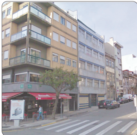
F _ THE YELLOW HOUSE Rua João das Regras 96
