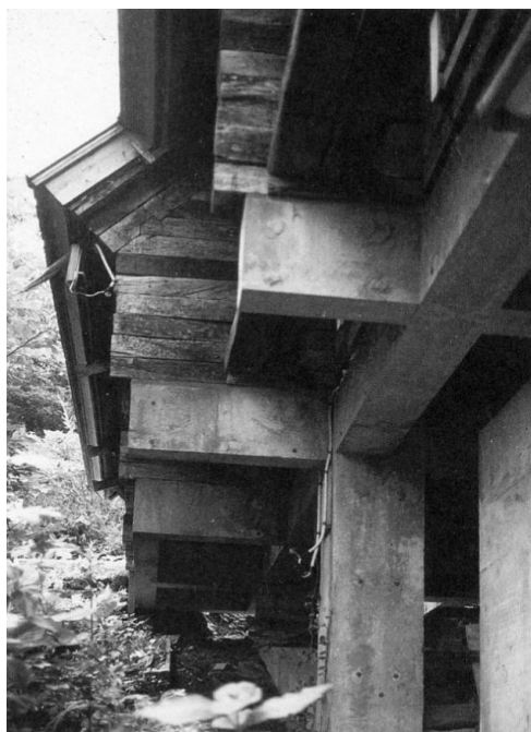
Fig.31 Esquerda: Railway House, fachada hasteal
