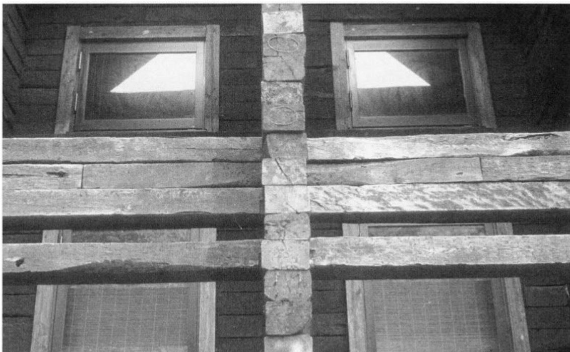
Fig.36 Railway House, detalhe
