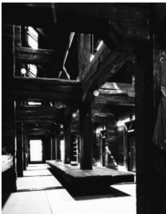
Fig.29 Esquerda: Railway House, vista interior
