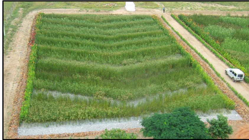
Figura 26 - Constructed Wetland . Fonte: https://www.biomatrixwater.com/msr-constructed-wetlands/
