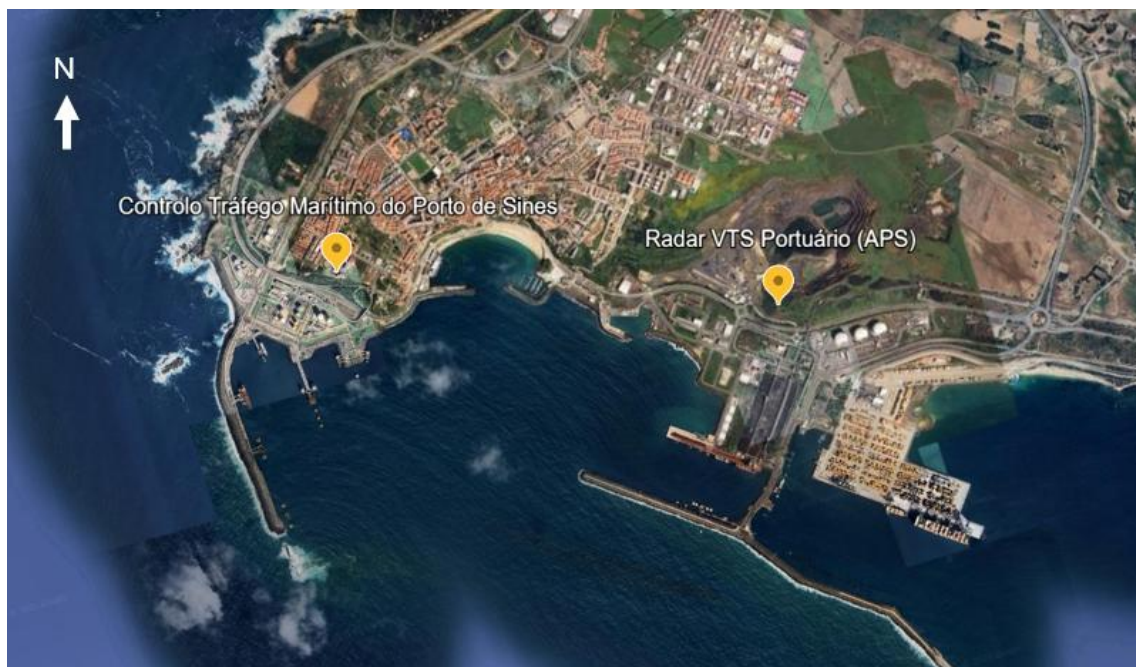
Figure 21- Possible Radar Antennas
