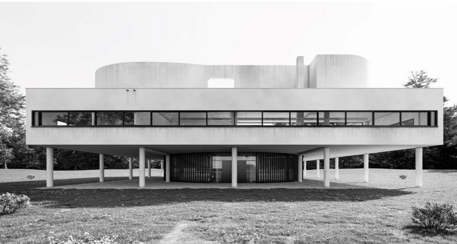
Figura 35 – Villa Savoye, Fachada principal
