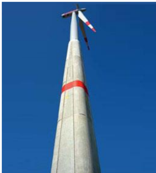
Figura 28 - Torre tubular (windpowermonthly, 27)
