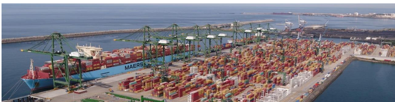
Figura 8- Terminal XXI - Sines
