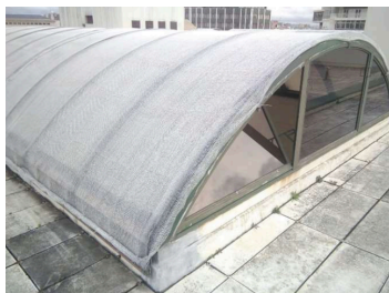
Figure 8 - Exterior of skylights with net
