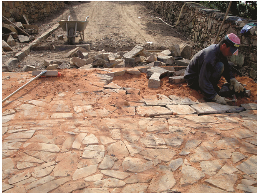
Figure 4. Execution of a traditional street pavement with schist stone under a GTAA Sotavento's project and works monitoring (Ribeiro, 2008a: 192).
