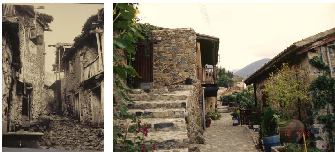
Fig.3 &4. Kakopetria settlement. Part of the settlement before and after restoration and rehabilitation. Source: Department of Antiquities of Cyprus.
