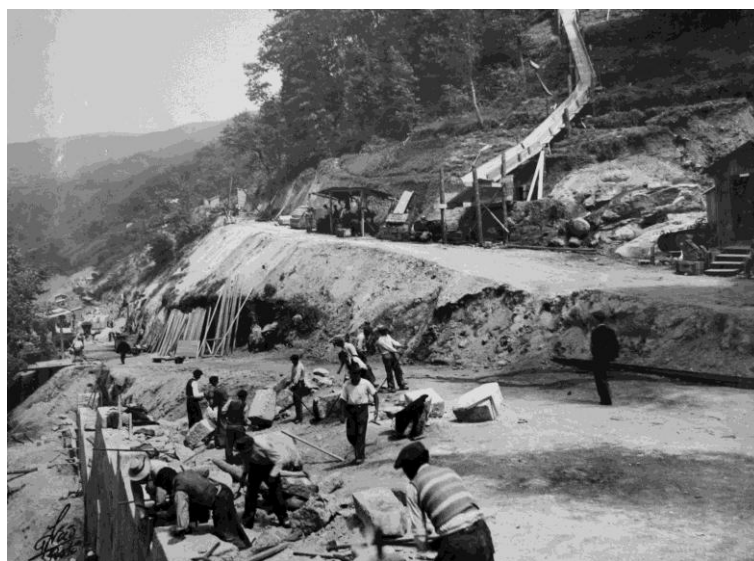
Figure 1. Access road to the hydroelectric Power station in Vila Nova, September 1948. Alvão photography ©, EDP archive, Porto.
