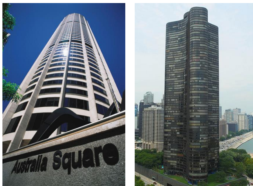
Figura 2.6 – Australia Square (Bird, 2011) e Lake Point Tower (River, 2010).
