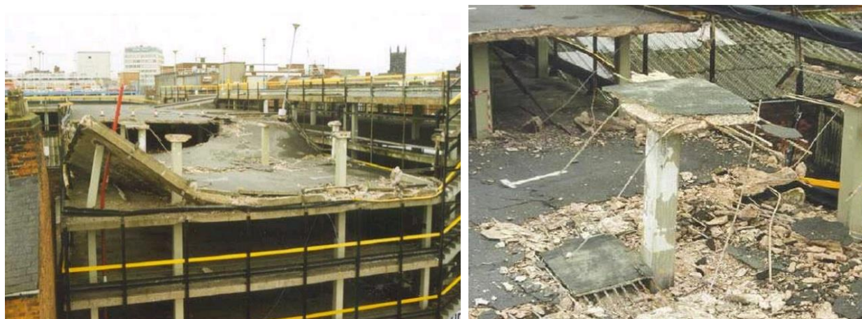
Figura 3.9 – Piper's row car park (Google, 2009).
