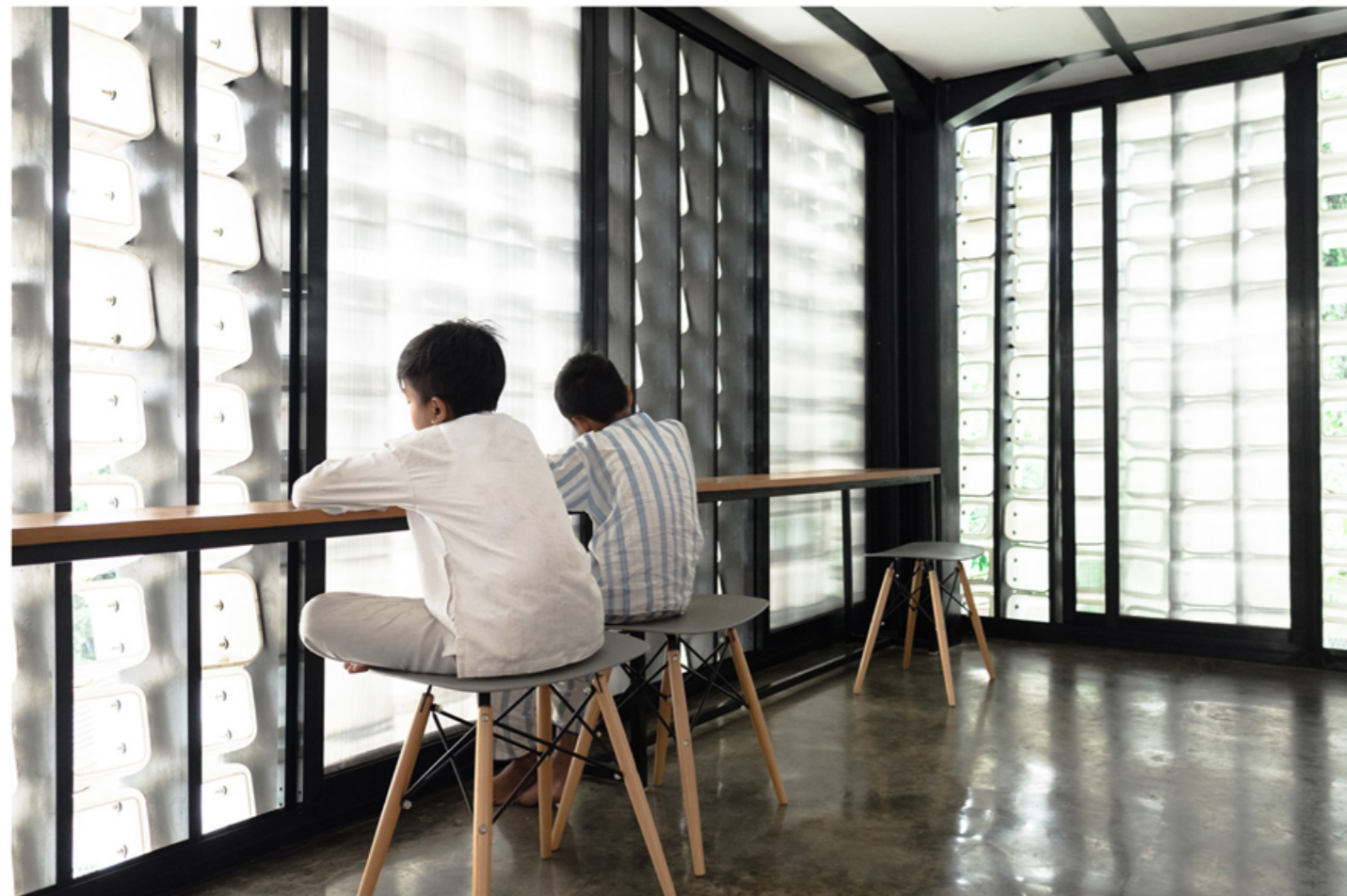
Figura 101 - Vista interior de parede semi-transparente (Archdaily, 2019)
