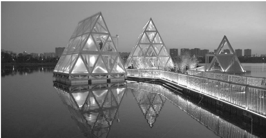
Figura 63 - MFS III, projeto Makoko Floating School do studio Nlé, na China (World Architecture, 2018)
