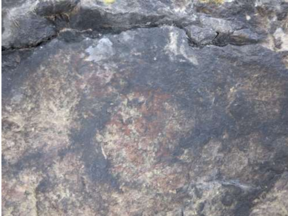
Figure 32 Impact of fire on the panels (Hipolito 2023).
