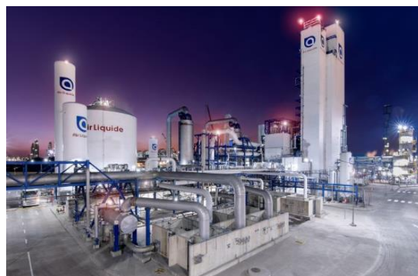
Figura 3- Air Liquide Engineering and Construction
