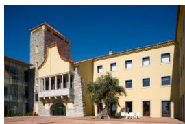
Hospital do Mar Fachada principal
