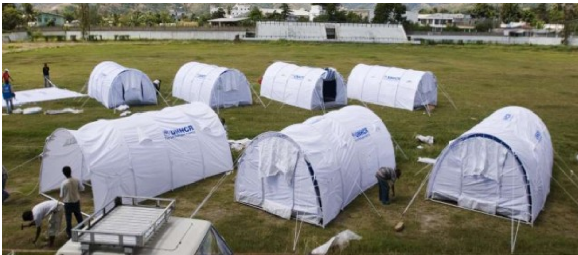
Fig. 50 - Montagem das tendas da UNHCR, as Lightweight emergency tent
