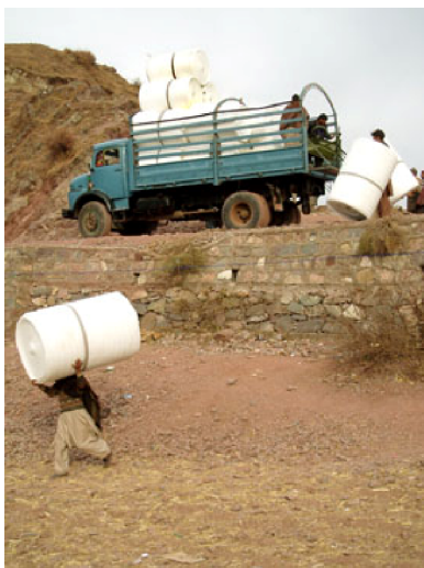
Fig. 102 - "winterization" of tents and structures: this foam is used as insulation in structures that are otherwise virtually useless.
