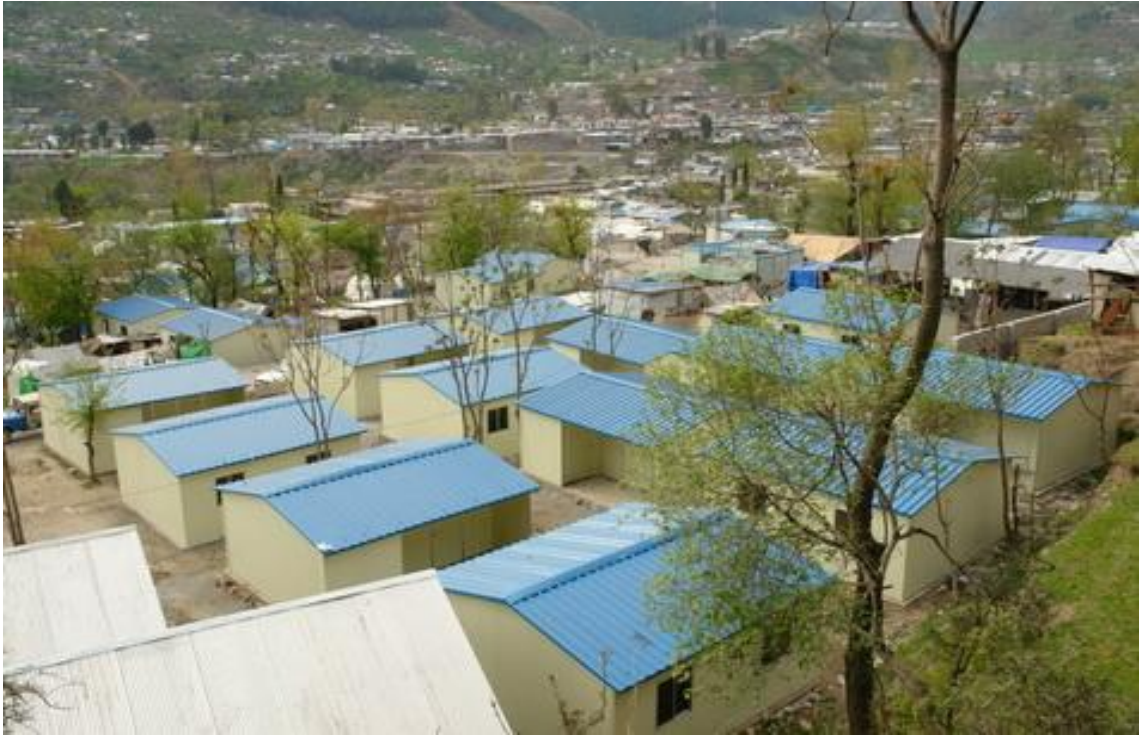
Prefab t-shelter from Saudi Public Assistance for Pakistan Earthquake Victims (SPAPEV) (Fonte: http://www.spapev.org/ )
