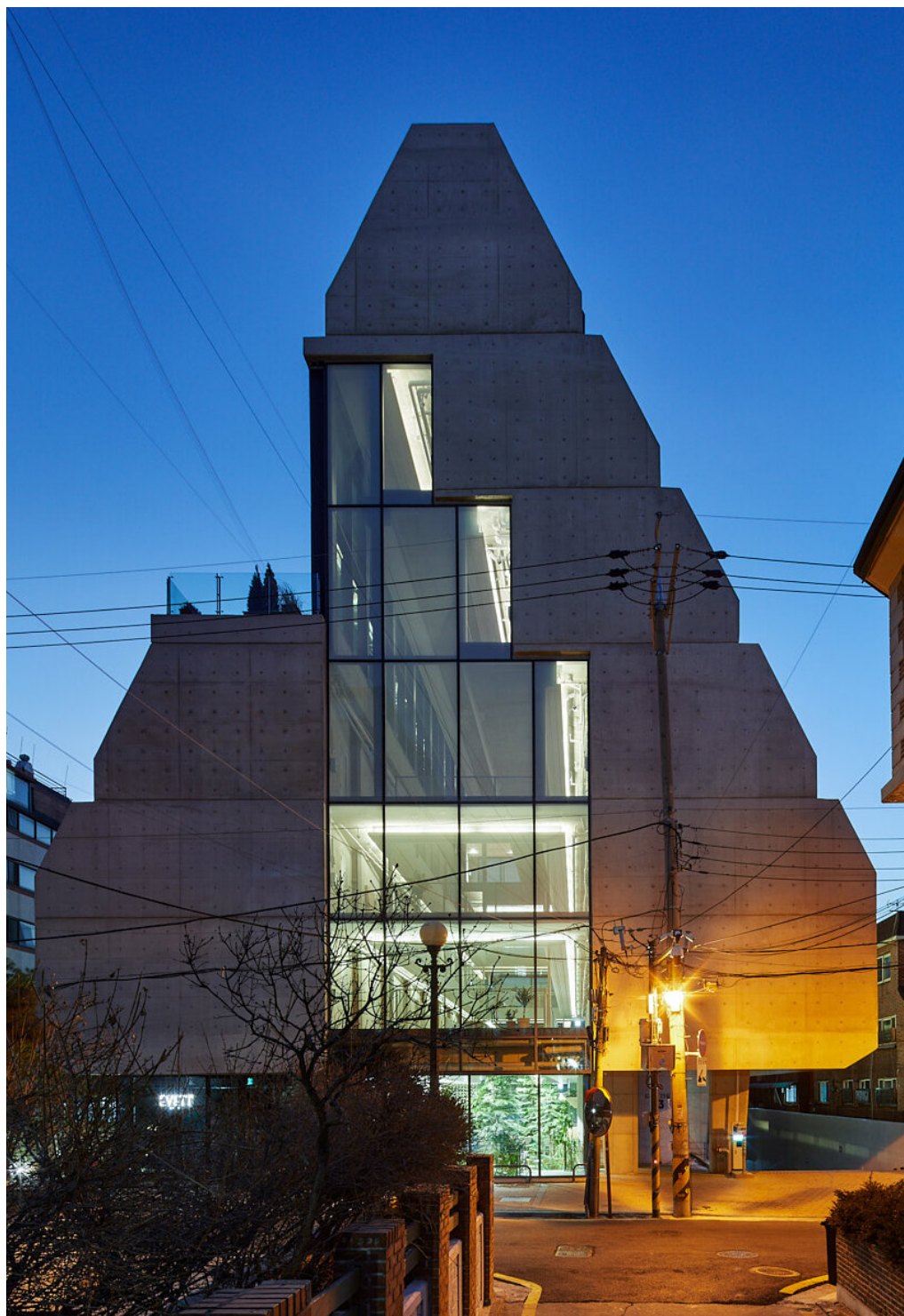
Fig. 62. Fachada Treehouse Coliving Apartments , Bo-DAA, 2018
