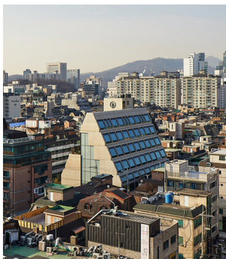
Fig. 60. Vista aérea Treehouse Coliving Apartments , Bo-DAA, 2018
