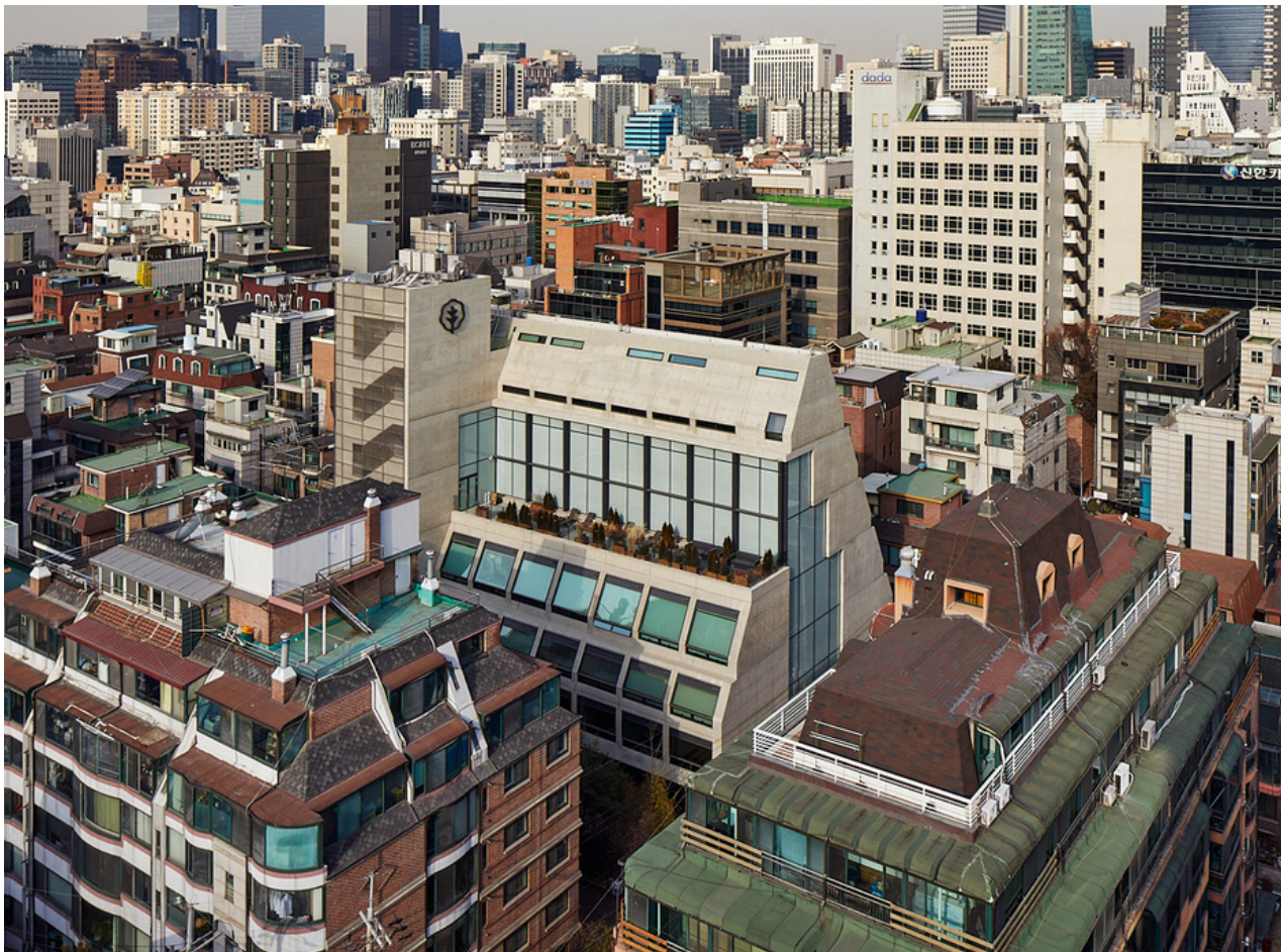
Fig. 55. Vista aérea Treehouse Coliving Apartments, Bo-DAA, 2018
