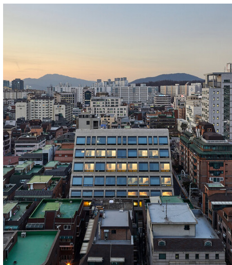
Fig. 59. Vista aérea Treehouse Coliving Apartments , Bo-DAA, 2018
