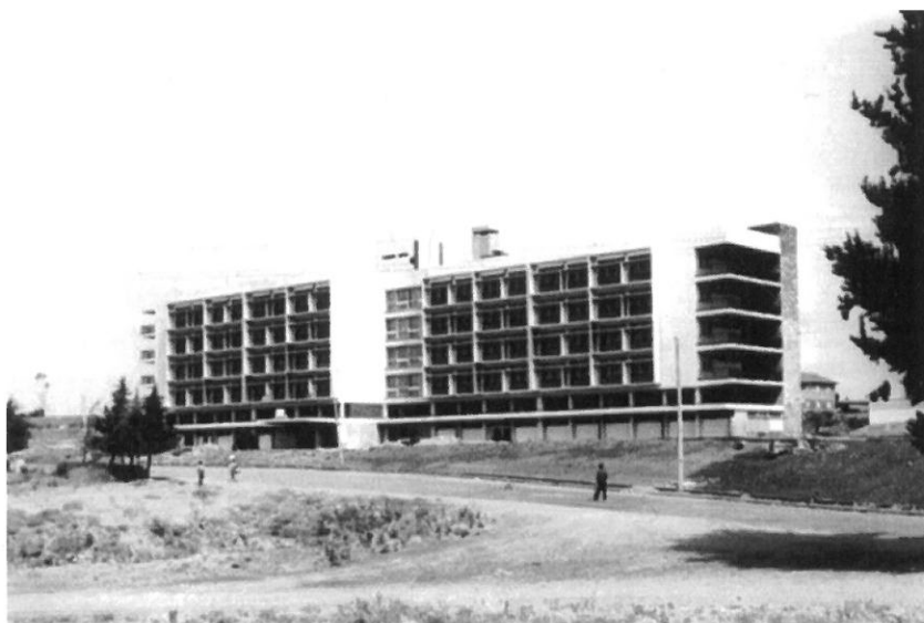
Fig. 36 – Vista Frontal do Hospital Regional de Bragança (1972)
