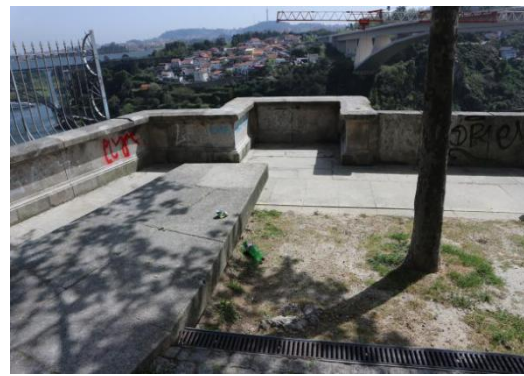
Fig. 36, River viewing wall
