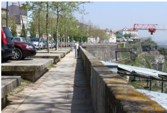
Fig. 35, Wall and tree bed area
