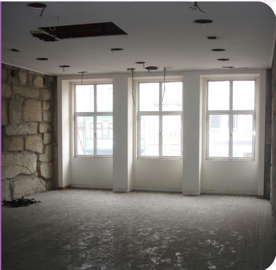
30. /31. view on the windows of the front elevation
