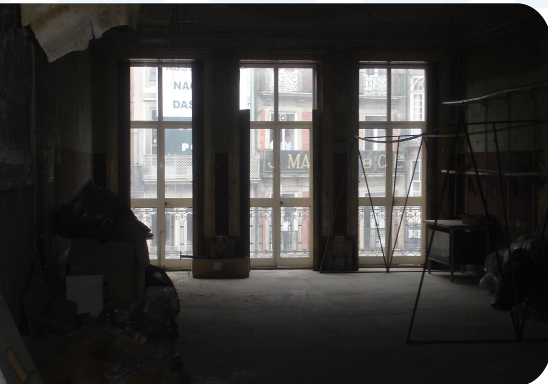
35. windows of the back elevation
