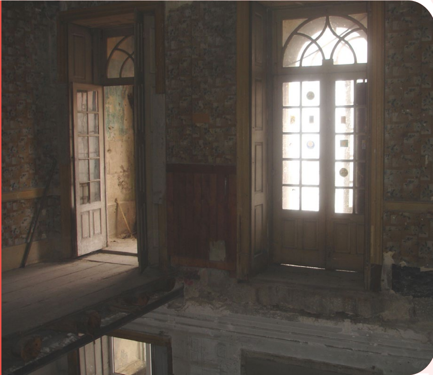
37. interior of the third floor
