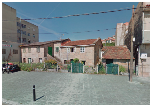
Figura 6 – antigua fábrica salazón de moaña - https://www.google.com/maps
