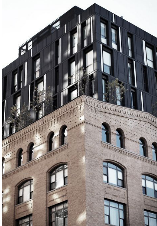
IMAGEM 77 The Porter House, SHoP Architects, Nova Iorque, América, 2002
