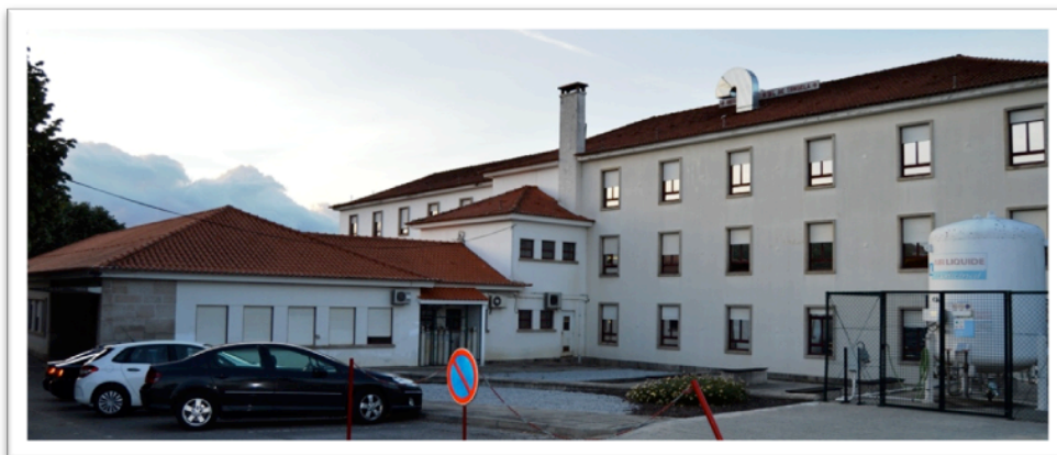
Figura 22 – Hospital Cândido de Figueiredo (Tondela) [38].
