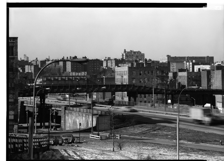
FIG. 01 Looking northwest at Third Avenue Elevated over Cross Bronx Expressway, 1974
