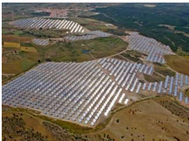
Figura 3.5 – Central fotovoltaica Amareleja ( Portal Energia, 2008)
