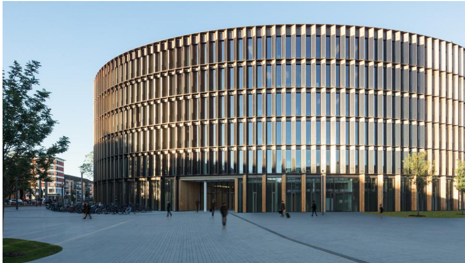
Fig. 44 – Camara Municipal de Freiburg ( https://www.dreso.ch/fileadmin/_processed_/d/5/csm_NVZ_Freiburg_c_HG_Esch_5e935dc259.jpg )
