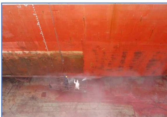
9 SBS-Same as previous photo where H.P. is progressing.
