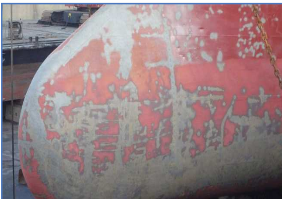
15 SBS-Bulbous area-Blasting work.
