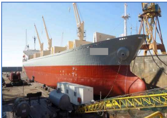
27 SBS- Paint work nearly completed.
