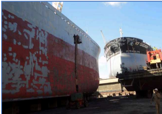
19 SBS.1st touch ups Hempadur 17630 Grey 11480 progressing.
