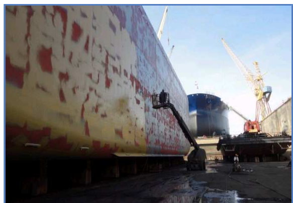
24 SBS-Hempadur 45182 Yellowish Grey progressing.
