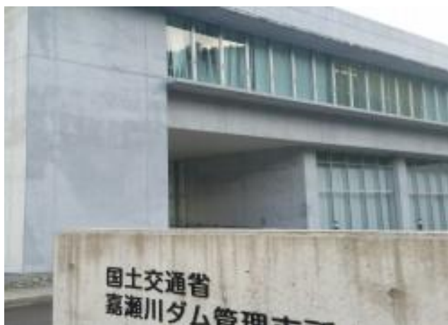
Figura 30: Edifício Kasagewa Dam, Northern Kyushu, Japão [PHOTOCATALYST COATINGS, 2014]
