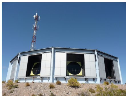
Figure 6: FD building at Los Leones during the day. Behind the building is a communication tower. This photo was taken during daytime when shutters were opened because of maintenance.
