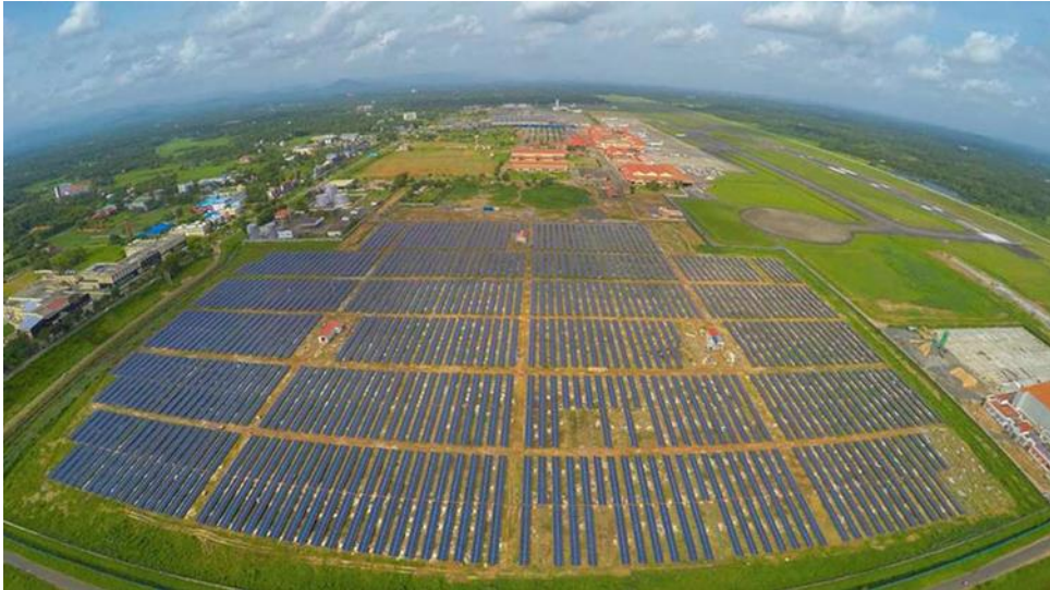
Figure 6 - Cochin International Airport solar power plant Source: (Akyüz 2018)
