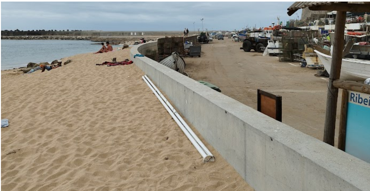
Figure 19: Beach (left side of the wall) spilling over to the fisherman's quarters (right side of the wall)
