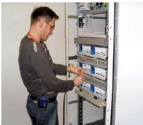
The mounting shelf goes inside the PMD Controller cabinet. There is room for 10 FCE Controller shelves per PMD controller cabinet, therefore a maximum of 20 FCE controllers per cabinet.
