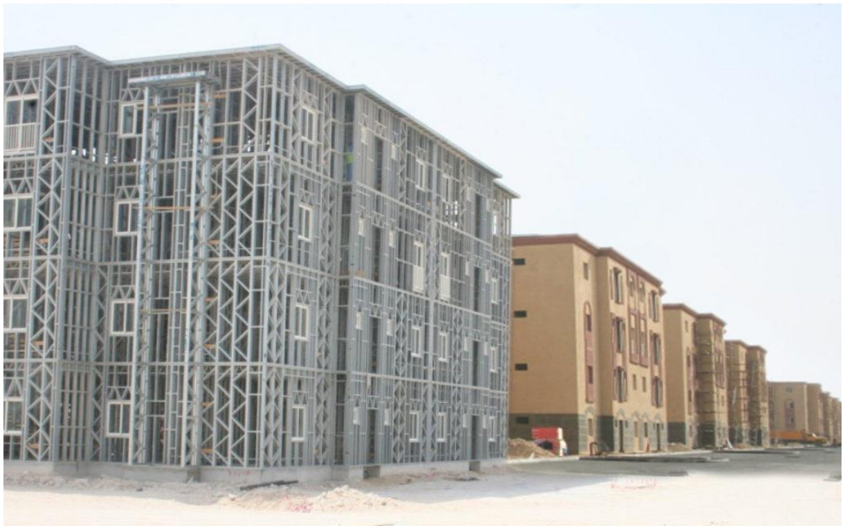
Multi Storey Apartment Block, Doha, Qatar (scottsdalesteelframes.com)
