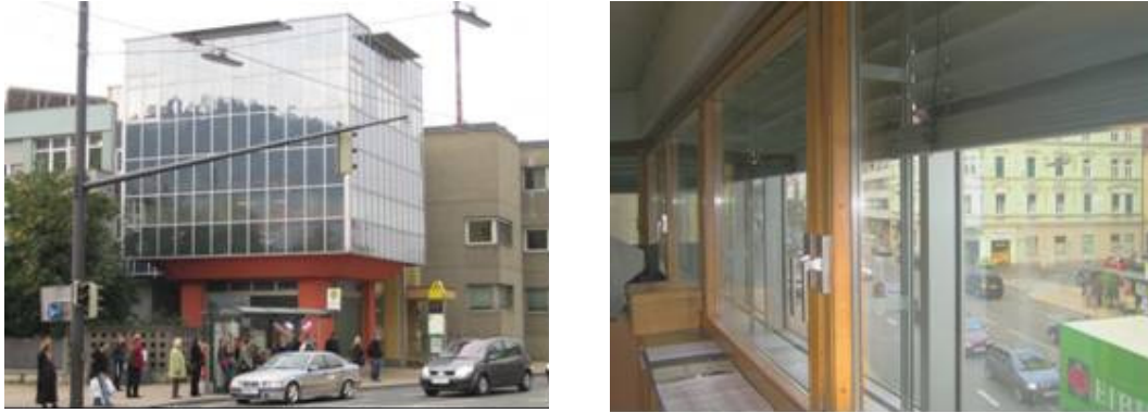
Fig. 1 Control room fire brigade Graz. The old wooden windows have been left as they were
