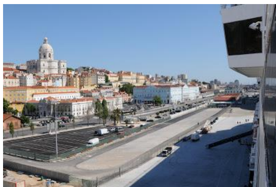
Fig. 27 - Terminal fluvial de Santa Apolónia (Google, 2016)
