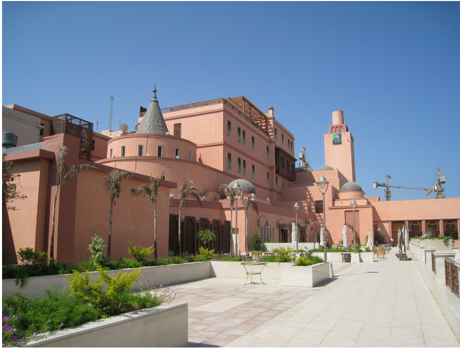
Figure 3. Hotel Uaddan in 2009, after a neo-moorish restoration: wooden musharabias and pergolas have been added. (Picture by the author, 2009)
