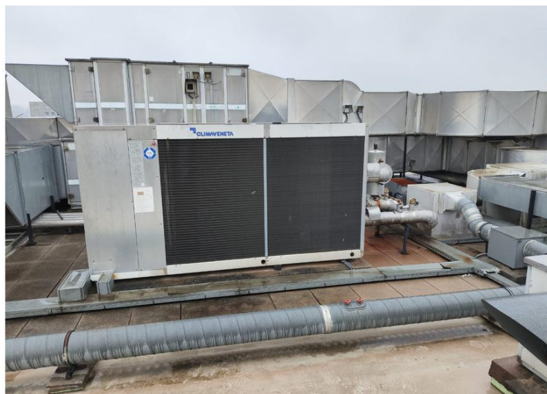
Figura 56 – Chiller CLIMAVENETA NECS 0452 B
