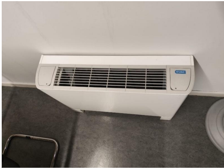
Figura 60 – Ventilconvector EVAC VC 34
