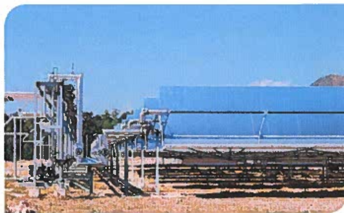
Figura 2 Refletores cilindro-parabólicos (Solarite CSP Technology GmbH [CC BY3.0 ( https://creativecommons.org/licenses/by/3.0/ )], via Wikimedia Commons).
