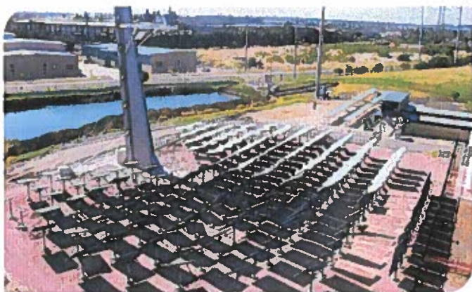
Figura 1 Sistema de recetor central (CSIRO [CC BY 3.0 ( https://creativecommons.org/licenses/by/3.0/ )]).
