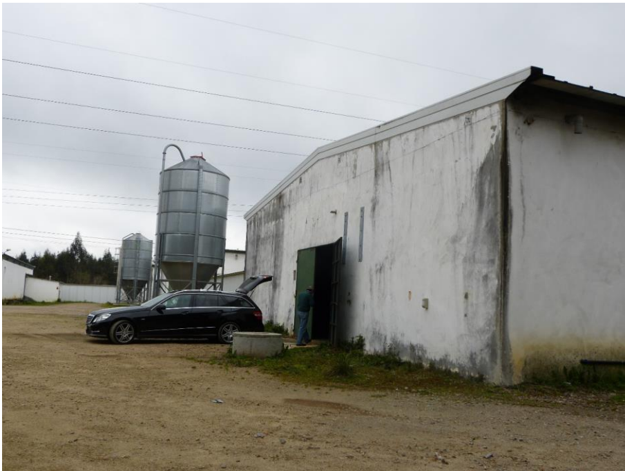
Picture 01 - Outside view of main entrance – no visible damage or signs caused by the fire.
