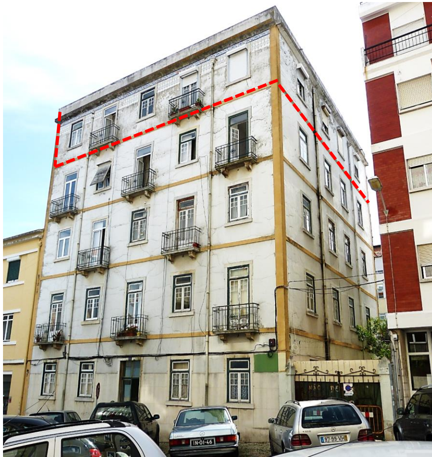
Picture 01 – View of the damaged building from the outside; to note that all the facades of the apartment in question – delimited by the red line – do not show any signs of damage.
