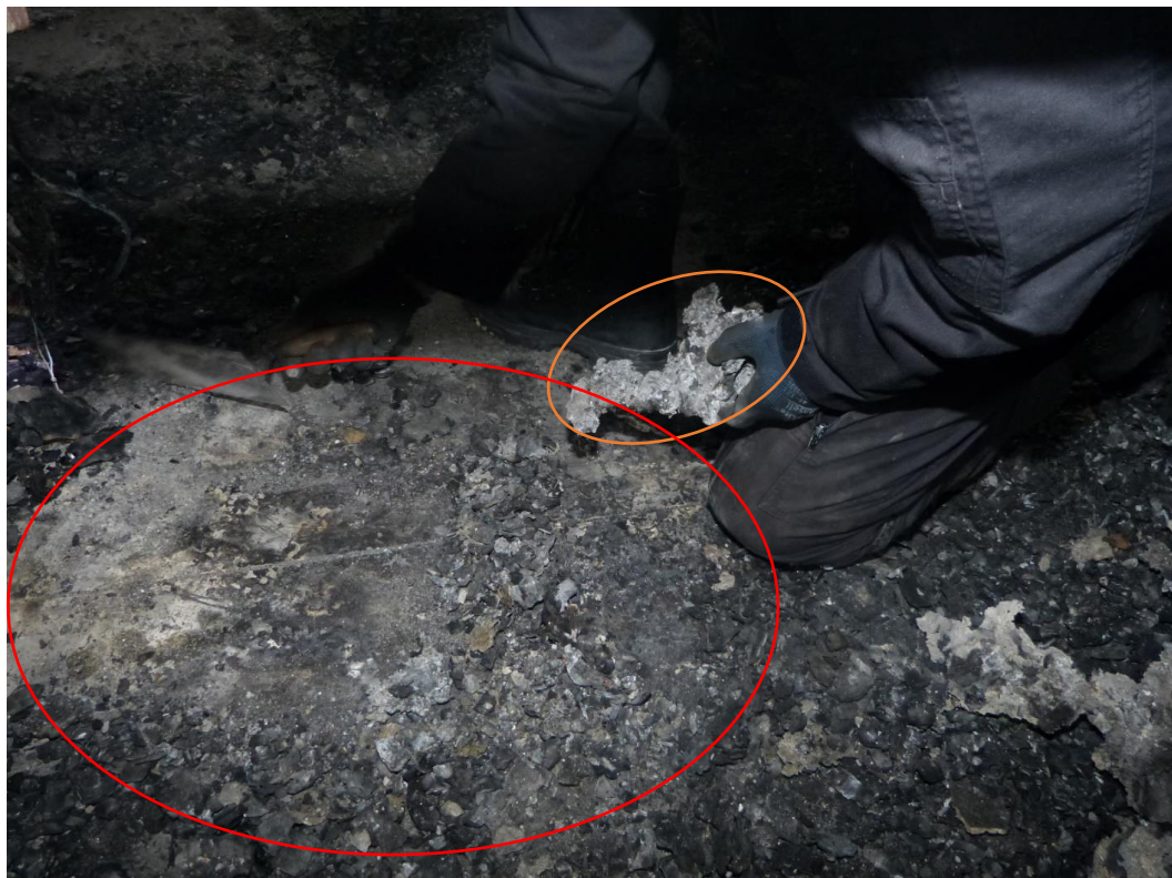
Picture 27 - View of floor area around tag #2 – completely melted bottom part of the engine (drop-down, orange ellipse); high levels of carbonization, no signs of ignitable liquid residues (red ellipse).
