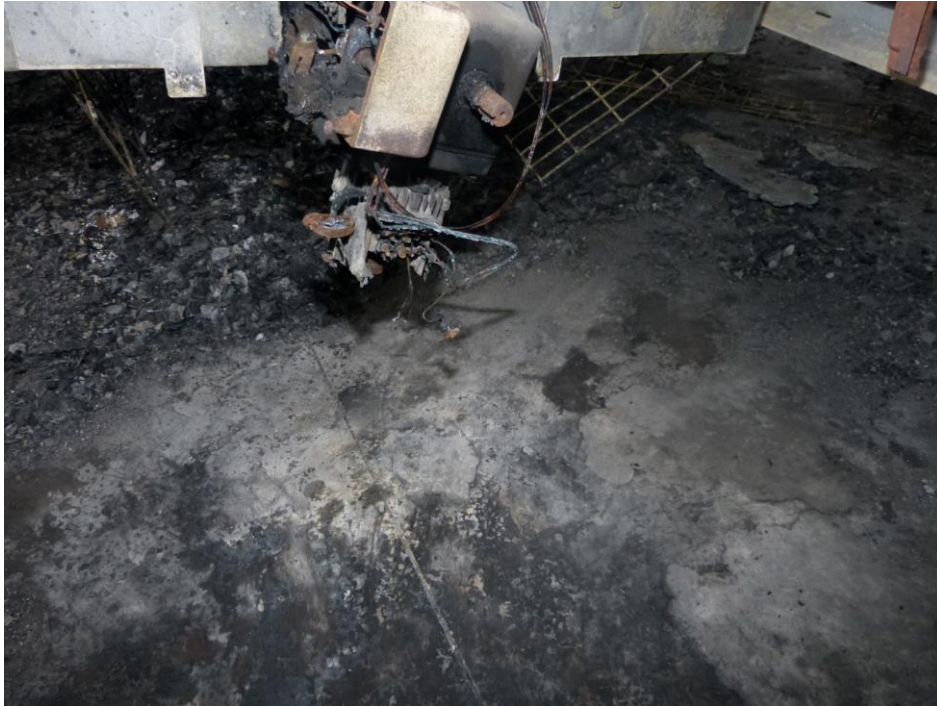
Picture 28 - View of floor area around tag #2 after removal of fire debris – no ignitable liquid residues visible.
