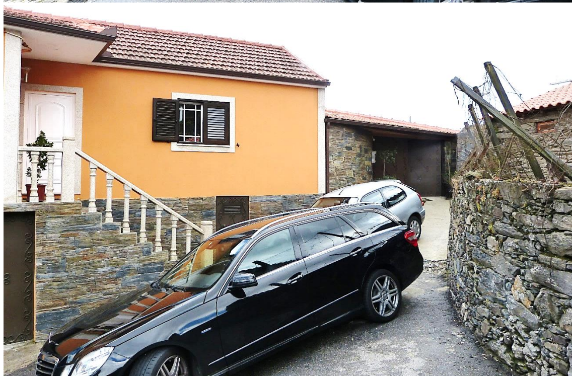
Picture 02 – No damages were observed in the other parts of the house.
