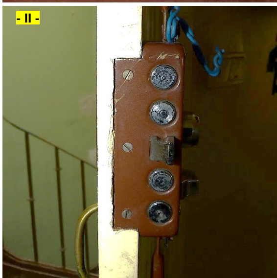
Picture 03 – Detailed view of the lock from the outside (I), the main frame (II) and the connecting part on the other side of the door (III) – no signs of forced entry.
