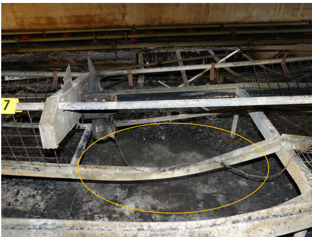
Picture 41 -View of floor underneath motor (tag#7) – no visible signs of presence of ignitable liquids (orange ellipse).
