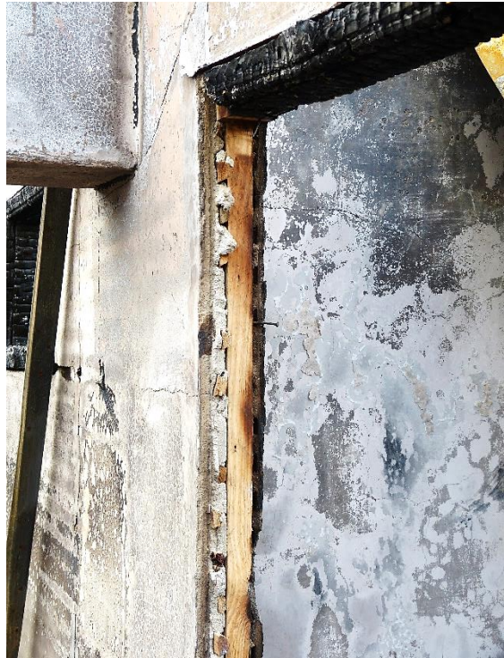
Picture 11 – Access door to the master bedroom. Major destruction of the doorjamb on the wall opposite to the window is observable.
