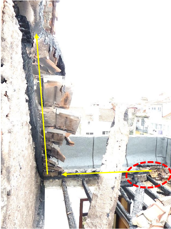
Picture 19 – Perspective of the area along the corner between the walls of the facades on the left side and the building's outer masonry.
