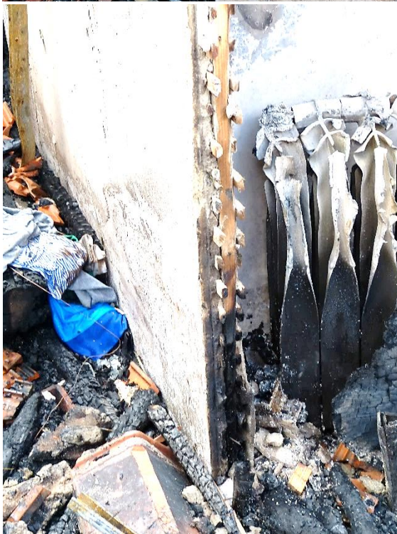
Picture 11 – Access door to the master bedroom. Major destruction of the doorjamb on the wall opposite to the window is observable.
