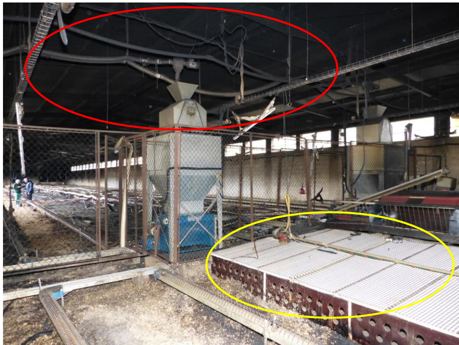
Picture 07 - Food supply machines – view from south to north, no discoloration or oxidation signs, chicken-houses almost intact (yellow circle) while ceiling shows soot deposition (red circle) signs of direct contact with flames and propagation on top, indicating point of origin further away from there.
