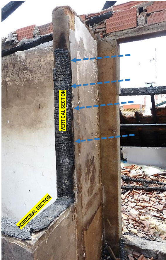
Picture 08 – Detailed view confirming the divergence of the damage present on the wooden balcony, identifying both directions of propagation of the fire in the sections of the horizontal and vertical profiles –red and blue arrows..
