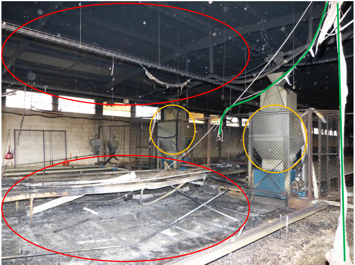
Picture 08 - Food Supply machines – View from north to south – soot depositions visible (orange circles), more on the right side (west) than left side (east), also major damage on floor (red bottom ellipse) due to completely absent chicken-house covers, metal bars showing high degree of soot deposition and oxidation and deformation, convective heat signs on ceiling (red top ellipse), residues of curtains on right of picture (green line), indicating that the fire was low on that part of the pavilion but had an upgoing trend when it reached the metal fence, directed more towards the right (west) side.
