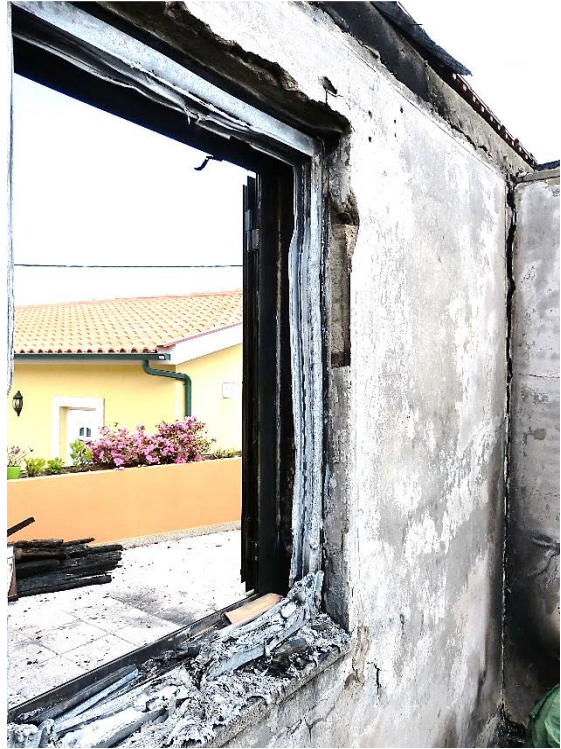
Picture 20 – Concomitantly with the observed on the outer face, the inner window had a greater concentration of damage on the left side –red arrows, consistent with exposure to heat for a longer time interval.
