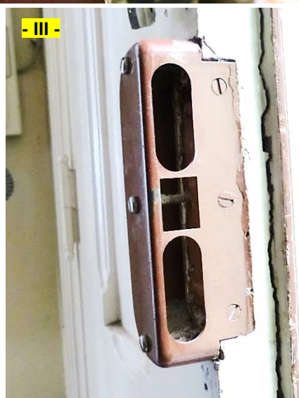
Picture 03 – Detailed view of the lock from the outside (I), the main frame (II) and the connecting part on the other side of the door (III) – no signs of forced entry.
