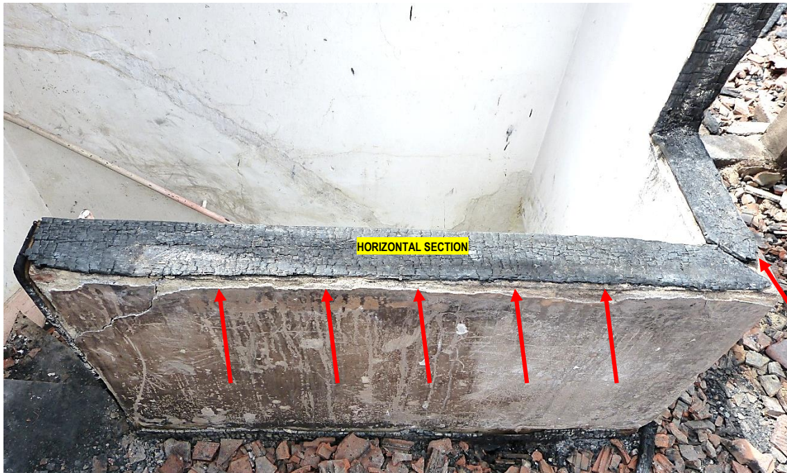
Picture 08 – Detailed view confirming the divergence of the damage present on the wooden balcony, identifying both directions of propagation of the fire in the sections of the horizontal and vertical profiles –red and blue arrows..
