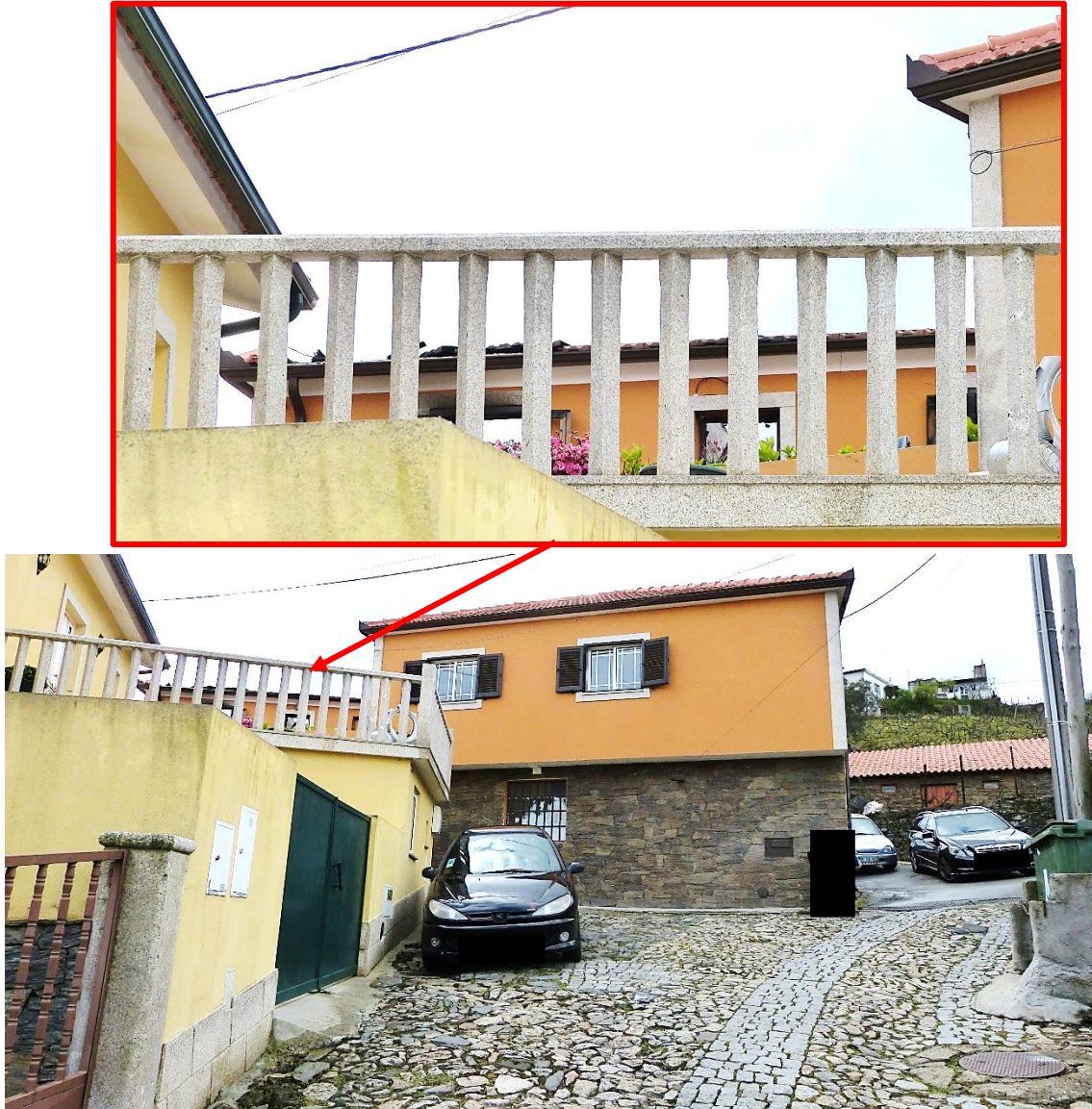
Picture 01 – Outer view of the house where the fire occurred: damages were only recorded in the area where the bedrooms were located.
