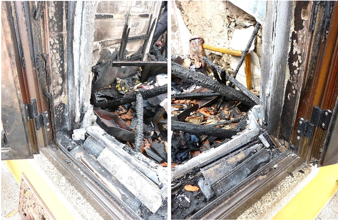
Picture 07 – Lower part of the window, confirming the direction of propagation.
